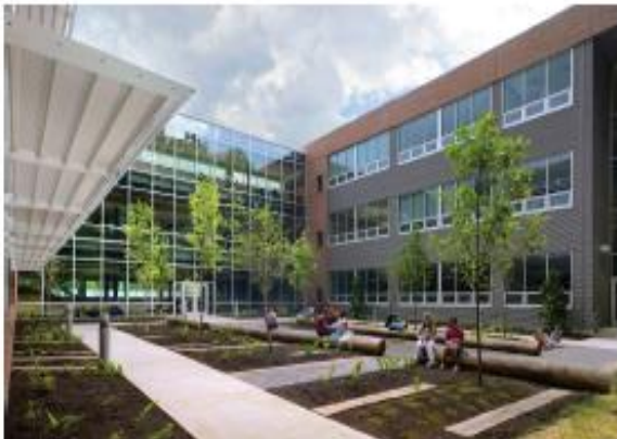
Above: Manassas Park Elementary School
